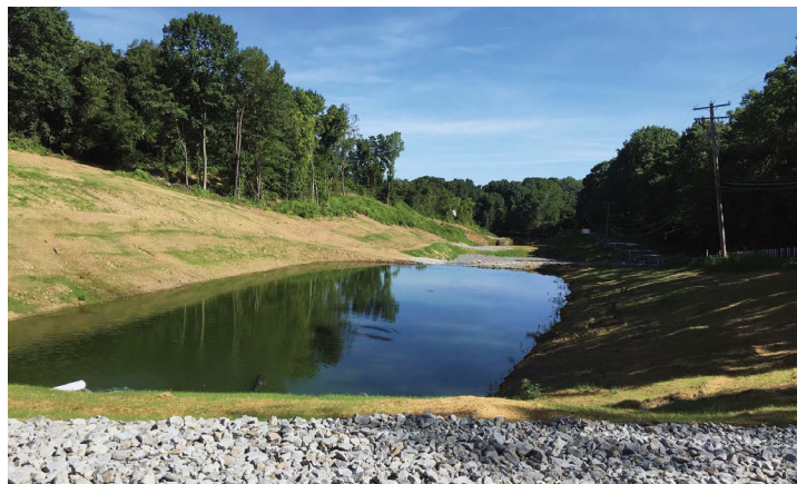
This series of ponds along Mahoney Road in North Fayette Township are now filtering acid mine drainage out of the Montour Run watershed.
